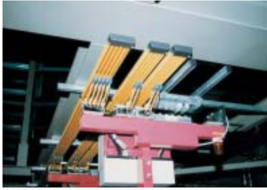
13 pole multipole conductor rail in 33 package distribution centres of the postal service (Post AG)
